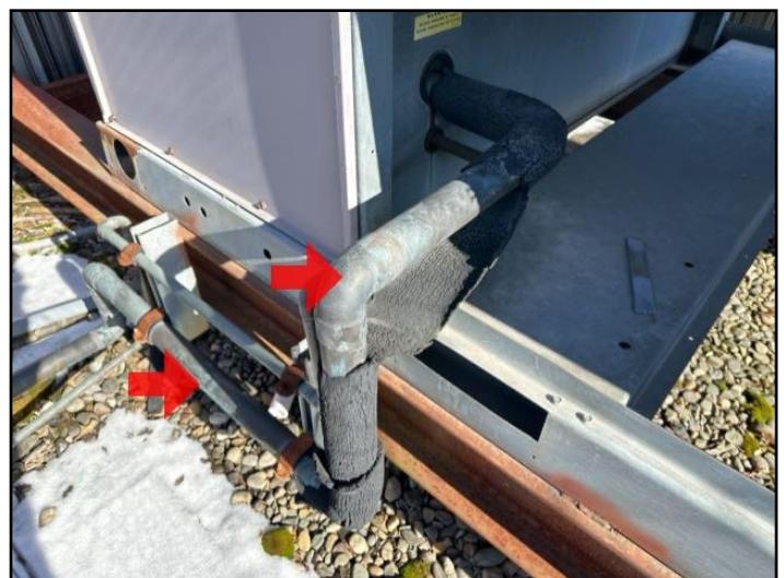
Insulation - missing
