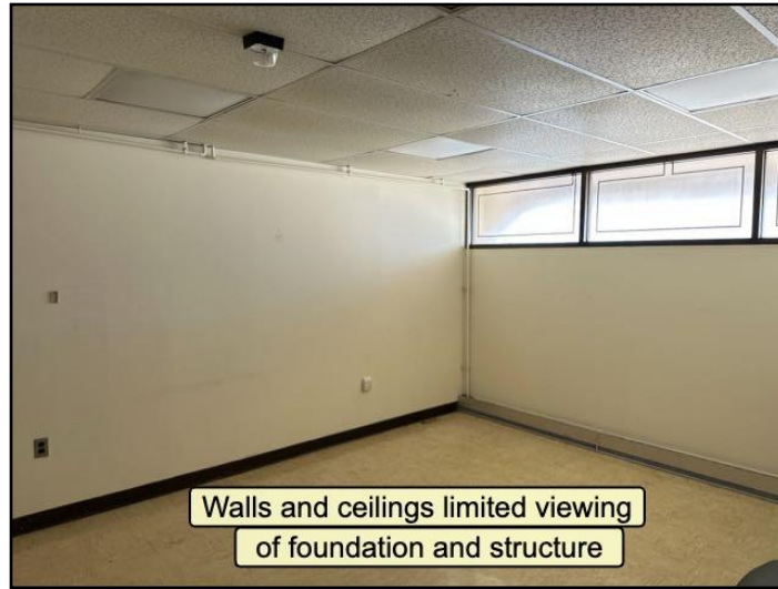
Basement finished walls and ceilings
