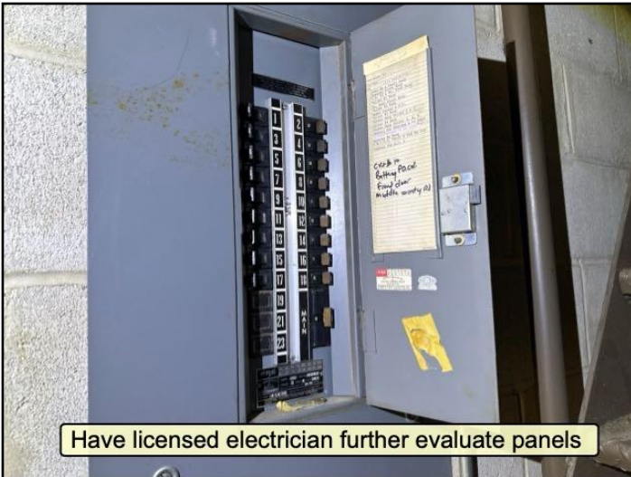
Old Federal Pacific electrical panels further evaluation recommended
