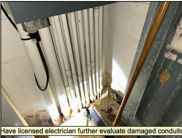
Conduit to electrical panel rusted in need of replacement
