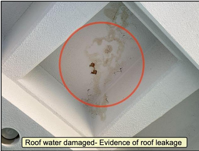
Water damage
