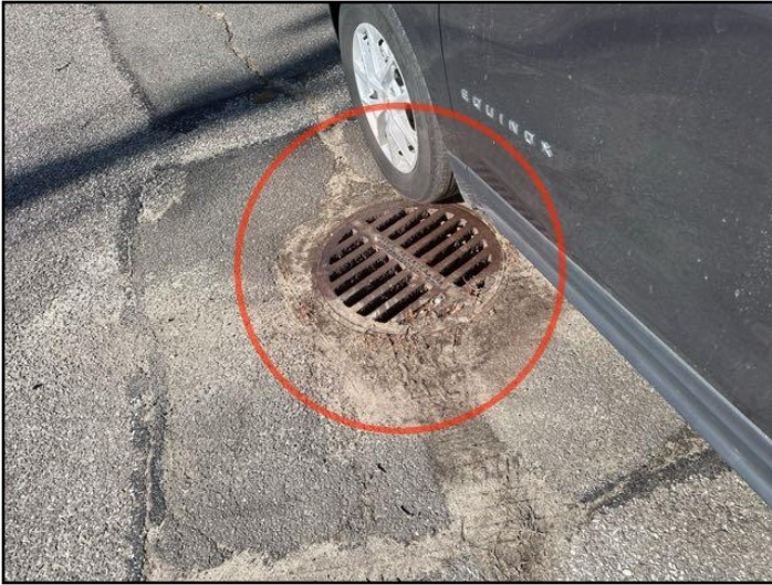
Keep outside drains clear of debris to...
