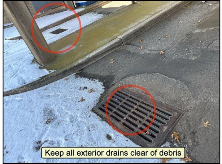
Keep outside drains clear of debris to...
