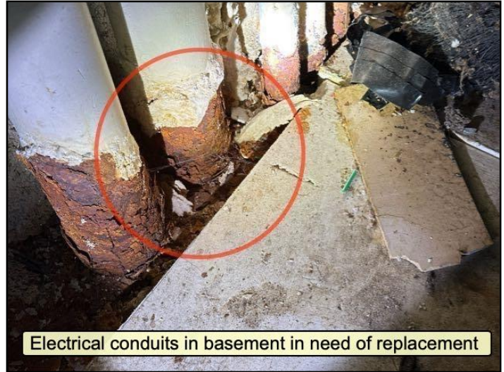
Conduit to electrical panel rusted in need of replacement
