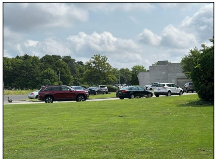
Missing parking lot lights
