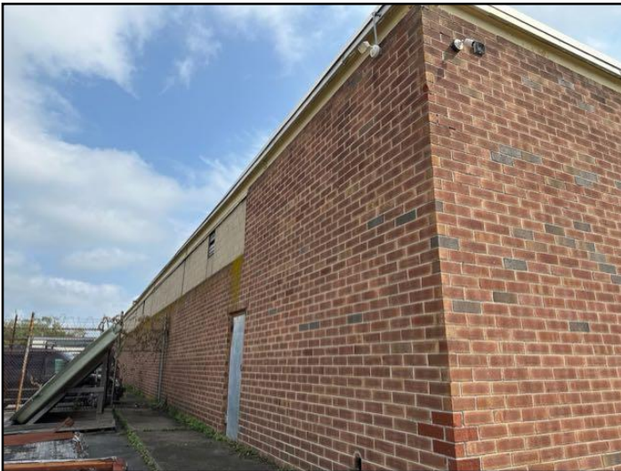
General view of structure
