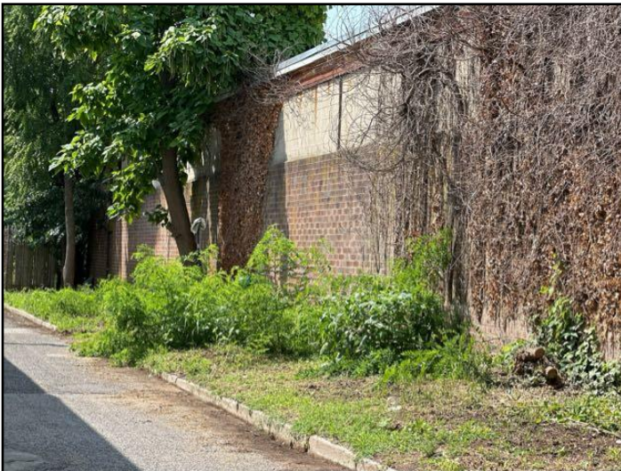
General view of structure
