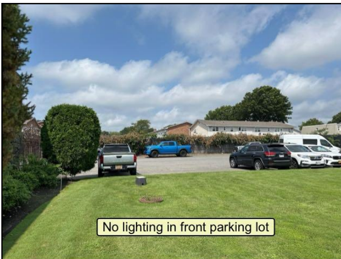
Missing parking lot lights
