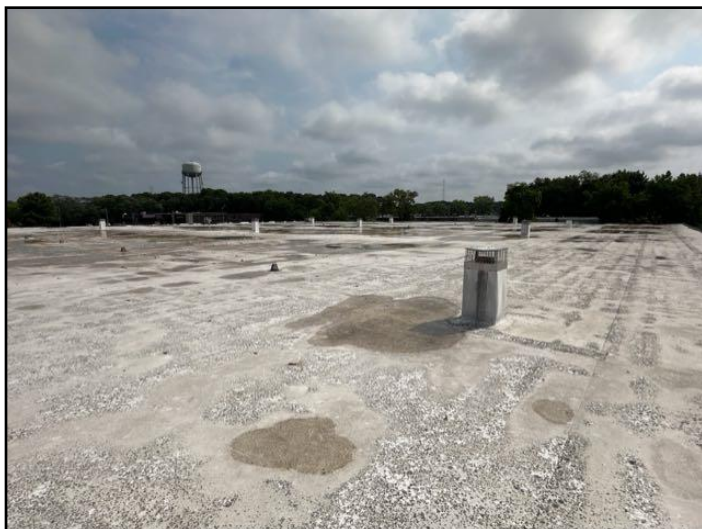
General view of Roof
