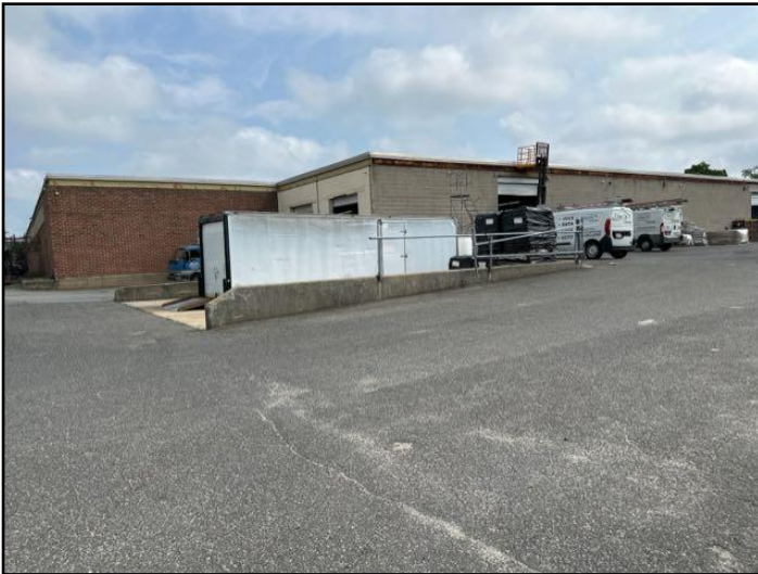
General view of structure
