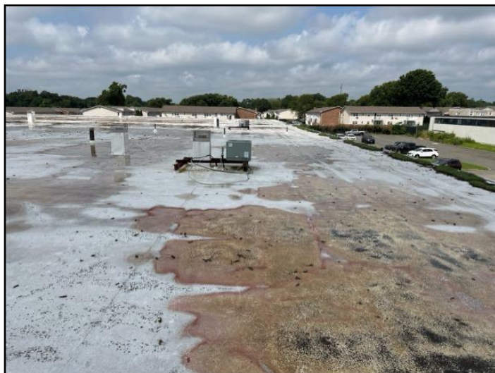
General view of Roof
