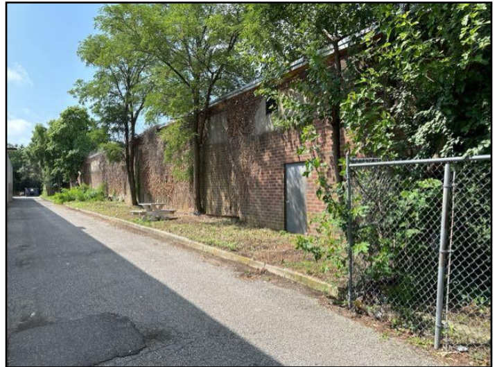
General view of structure
