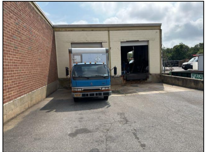
General view of structure
