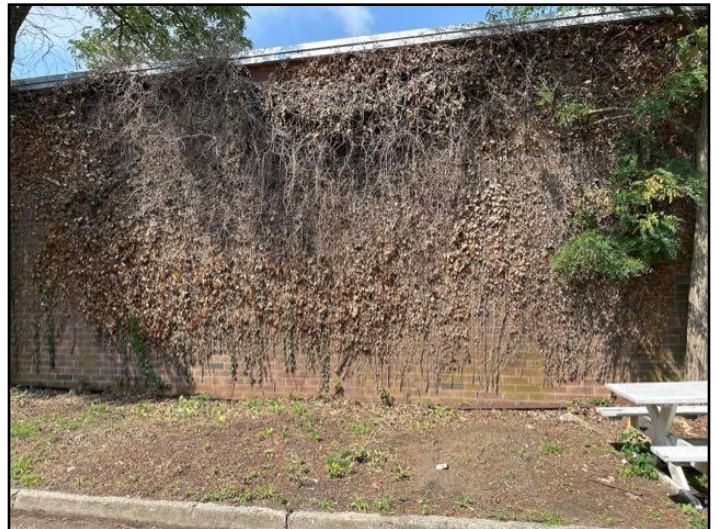
General view of structure
