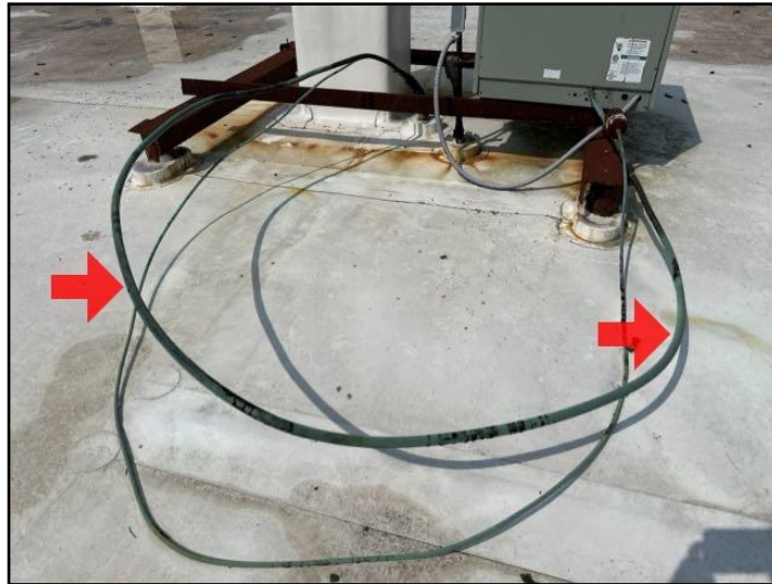
Insulation - missing
