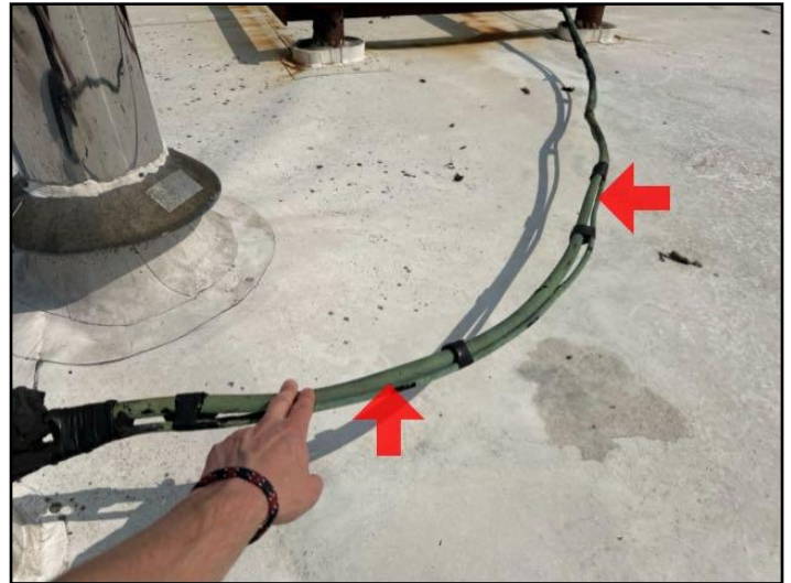
Insulation - missing
