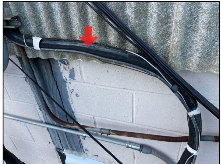
Insulation - missing
