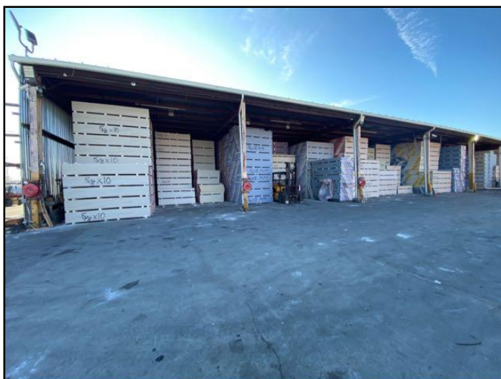
General view north side
