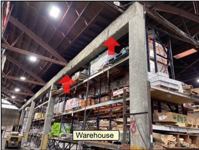
General view of structure
