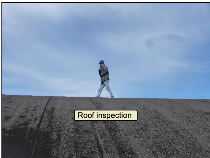
By walking on roof
