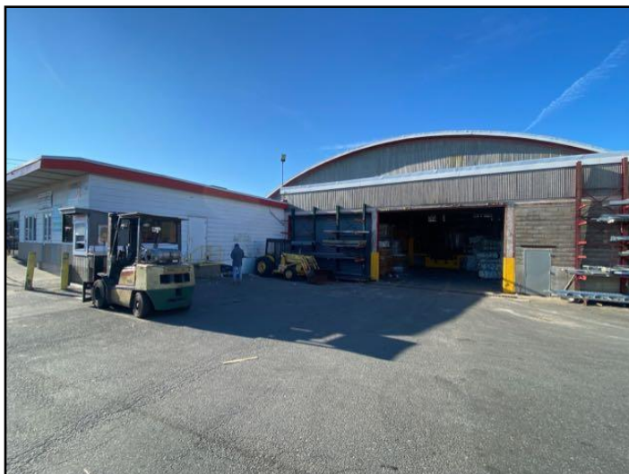
General View East Side
