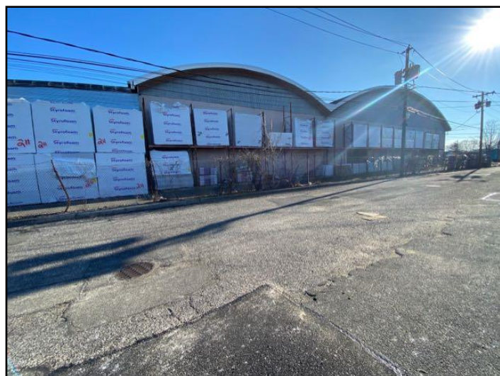
West side of building
