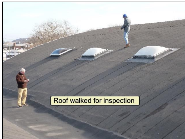
By walking on roof
