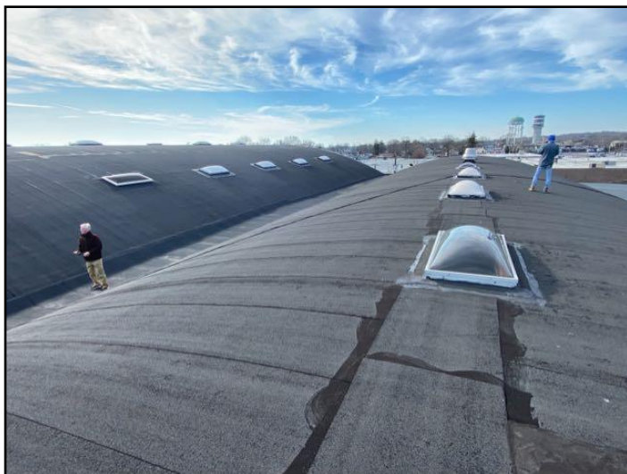
General view of Roof
