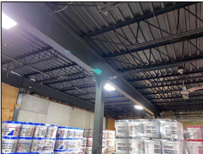
General view of structure
