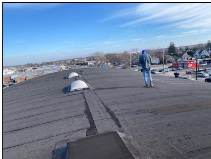
General view of Roof
