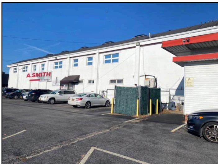
South side of building
