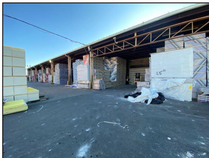
General view north side
