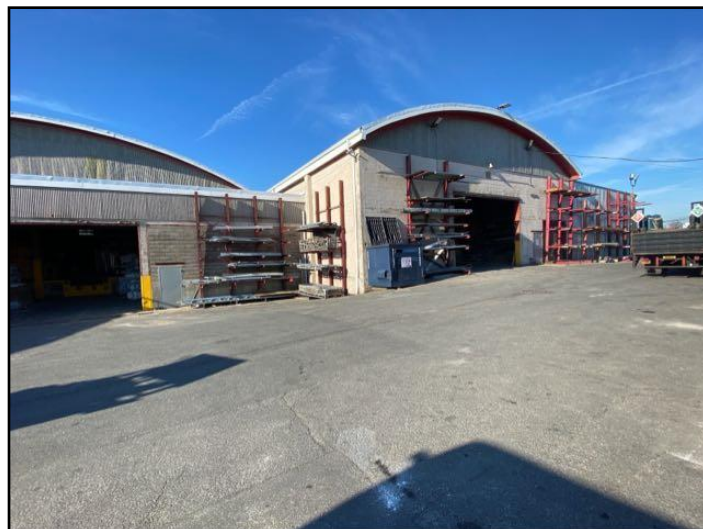
General View East Side
