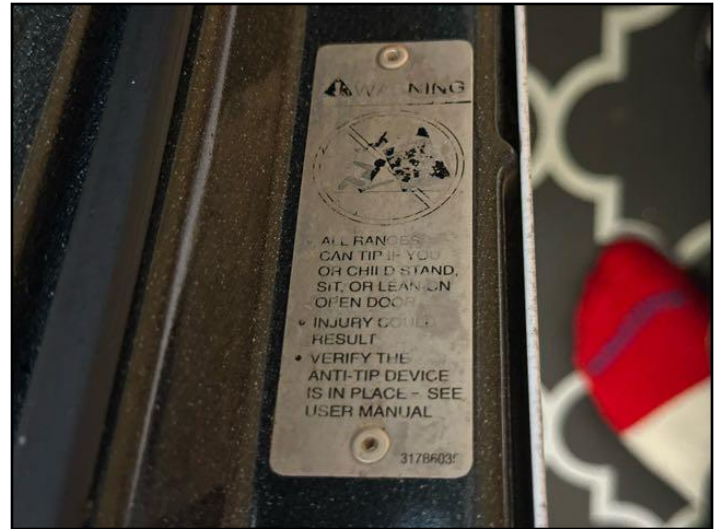
Anti-tip device missing
