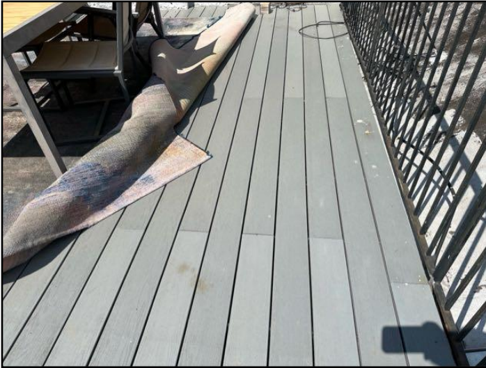
Deck covering roof
