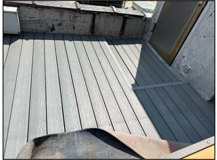
Deck covering roof
