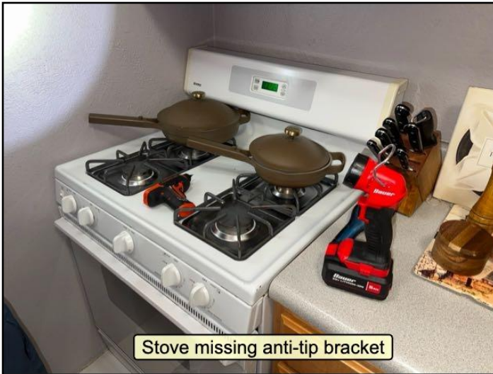
Anti-tip device missing
