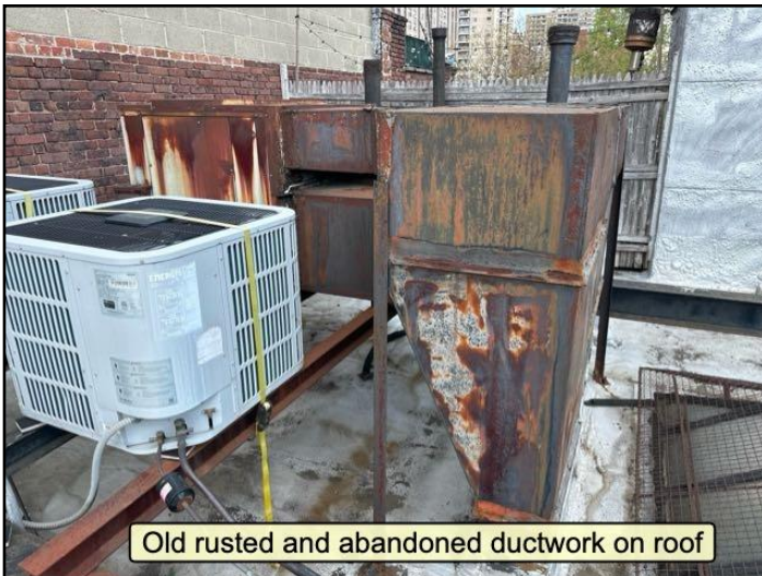
Older uninsulated ducts
