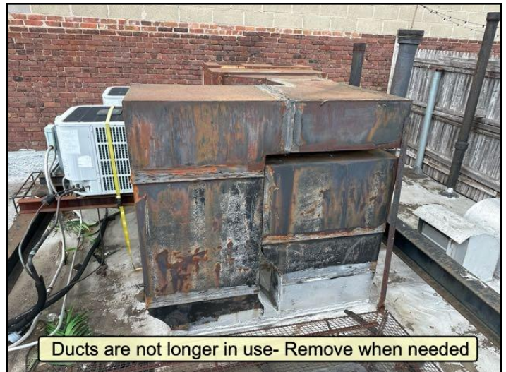
Older uninsulated ducts
