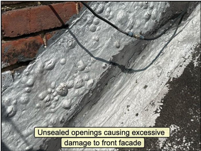
Prior temporary repairs
