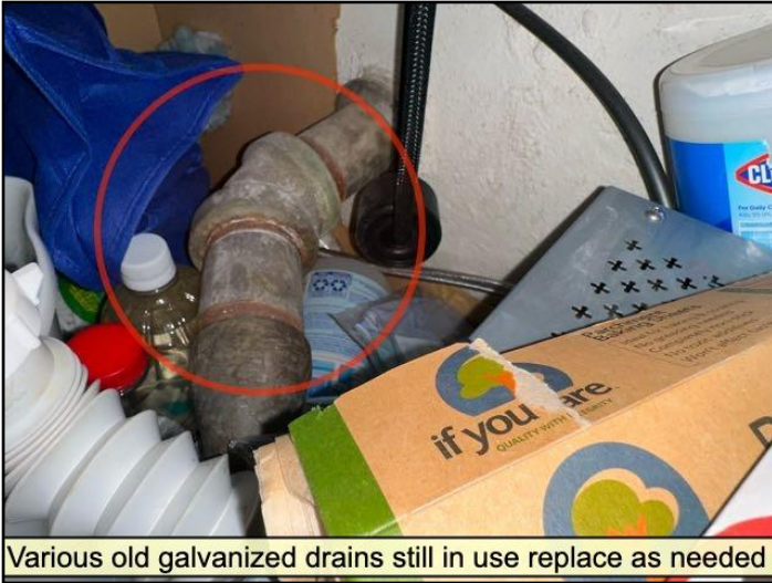
Old galvanized drains
