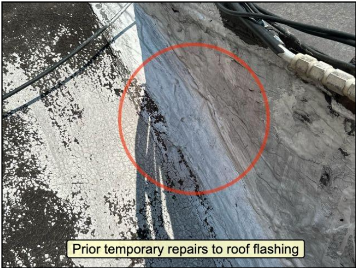
Prior temporary repairs
