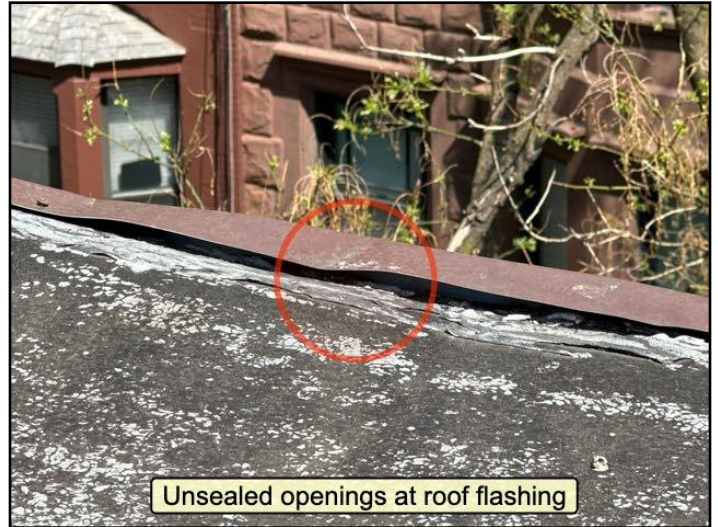
Replace when re-roofing
