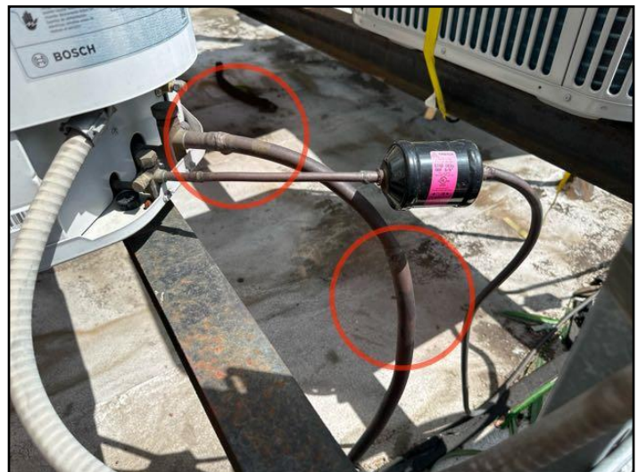
Insulation - missing
