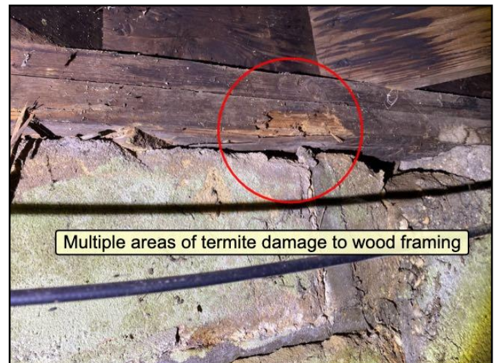
Termite damage
