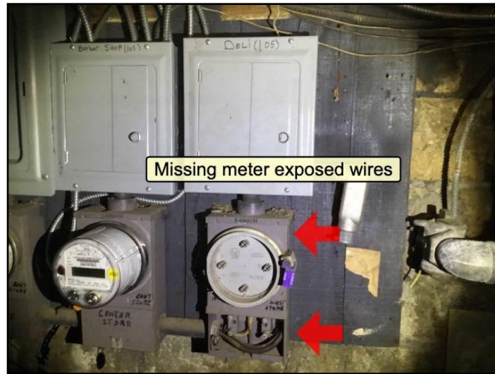
Unprotected openings
