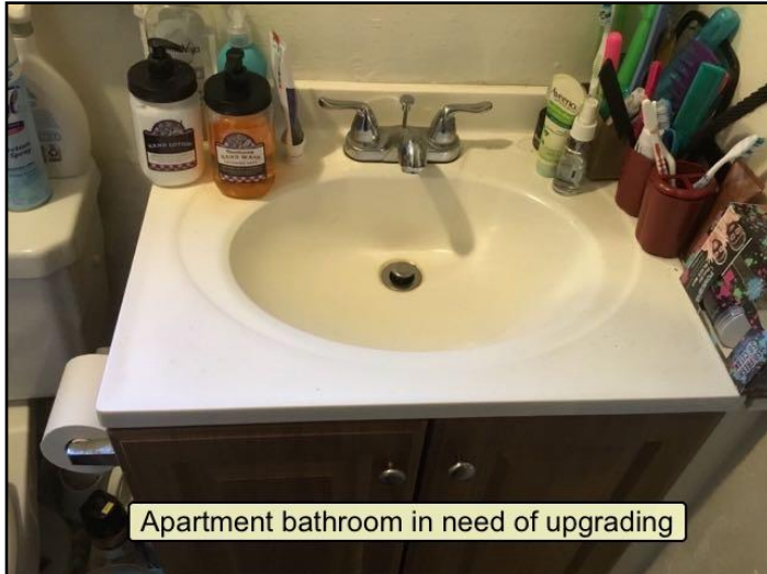
Bathroom in need of upgrading. Recommend...
