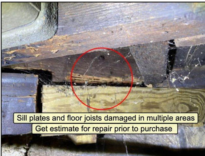
Termite damage
