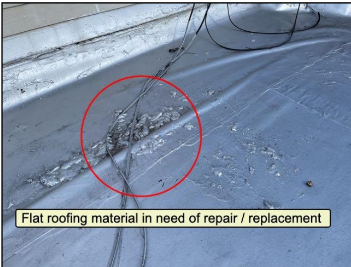
areas of rolled roofing material wrinkling and blistering
