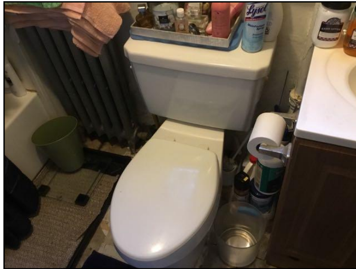
Bathroom in need of upgrading. Recommend...
