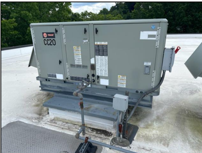
Trane- Packaged Rooftop Unit (RTU)
