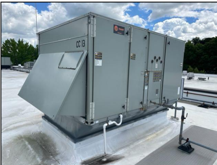
Trane- Packaged Rooftop Unit (RTU)
