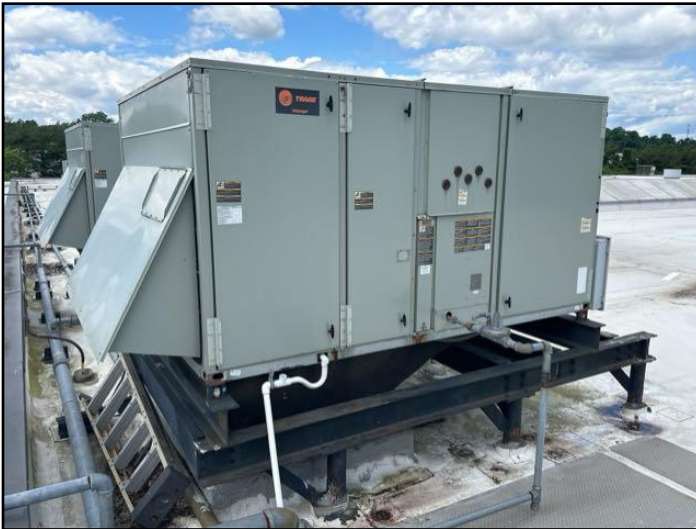
Trane- Packaged Rooftop Unit (RTU)
