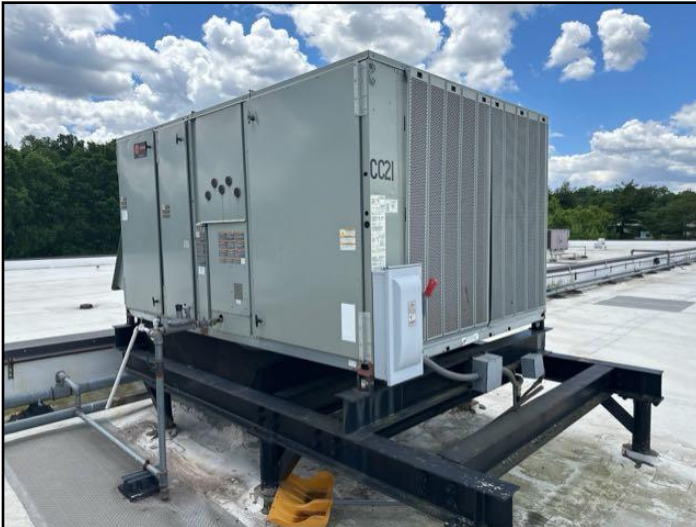
Trane- Packaged Rooftop Unit (RTU)
