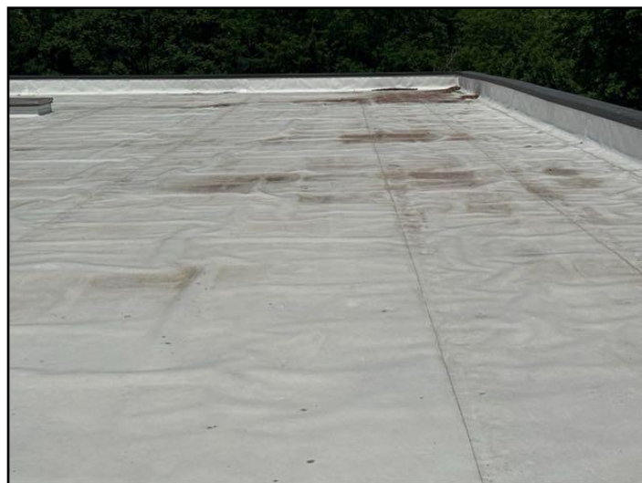
General view of Roof
