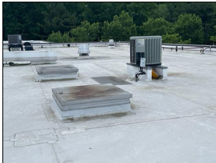
General view of Roof
