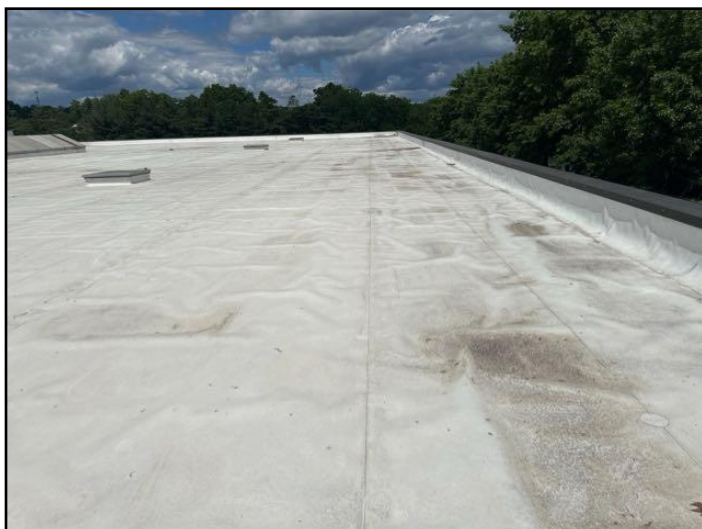
General view of Roof
