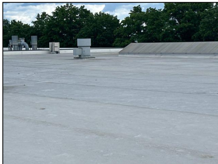
General view of Roof
