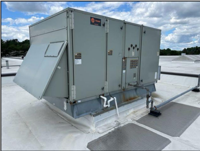
Trane- Packaged Rooftop Unit (RTU)
