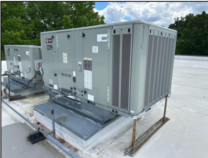
Trane- Packaged Rooftop Unit (RTU)
