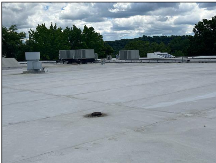
General view of Roof
