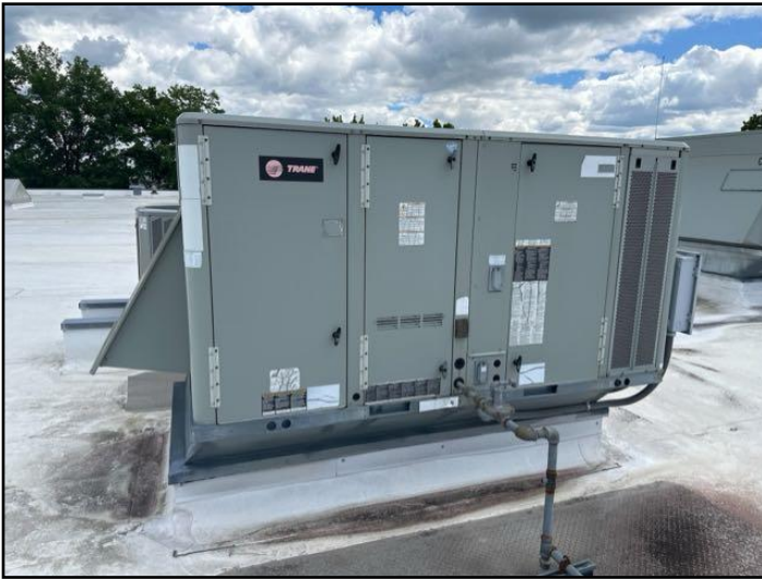
Trane- Packaged Rooftop Unit (RTU)
