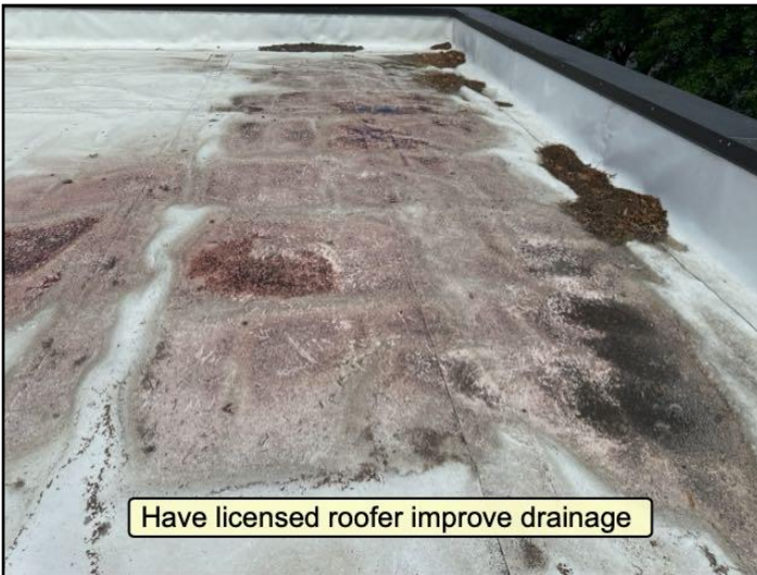
Ponding and puddling in various location
